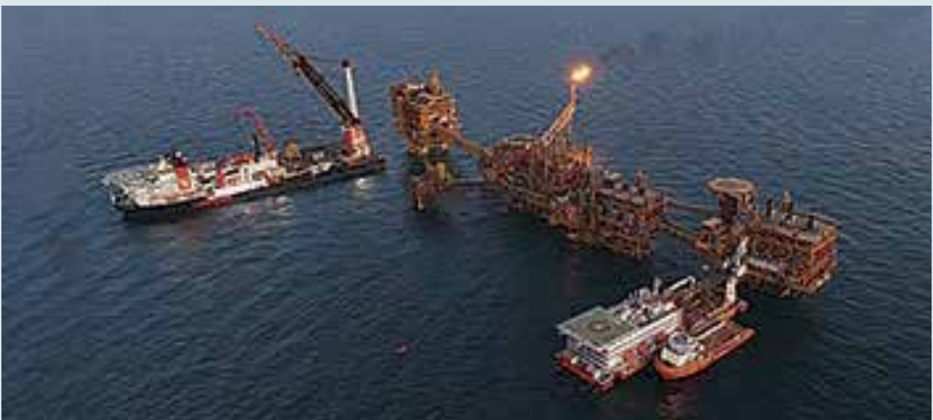
Offshore Crane, Allianz Intrepid (Accommodation Barge)
