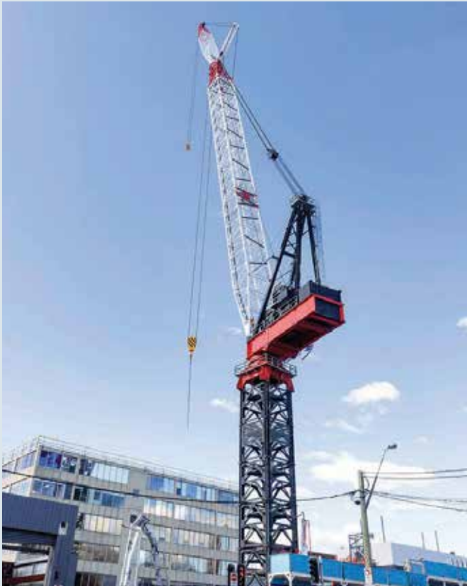
Tower Crane with Superfly, Sydney Metro Station, Australia
