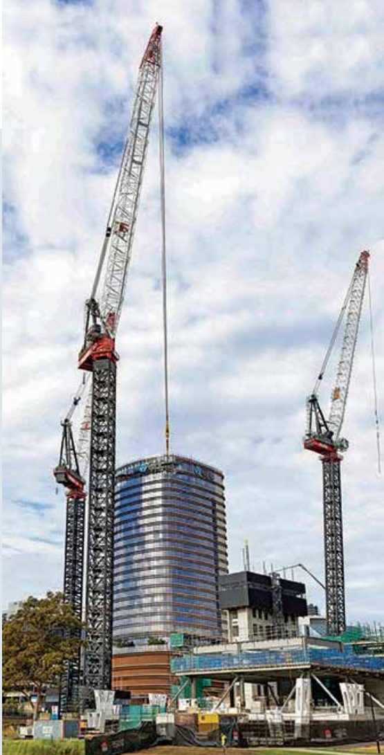
Tower Crane, Powerhouse Museum, Australia
