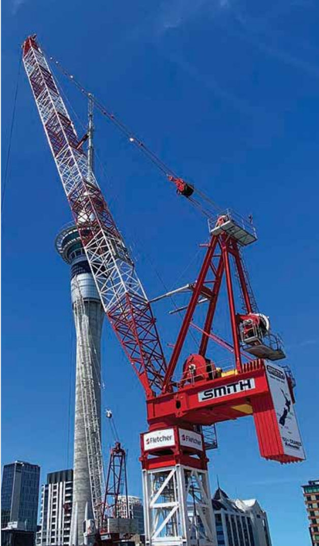
Tower Crane, New Zealand International Convention Centre, New Zealand
